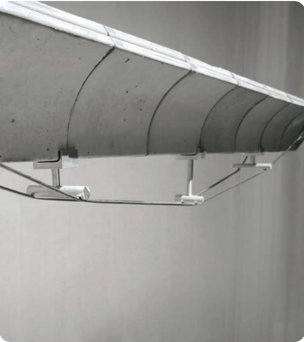
Steel tie rods on concrete bridge
