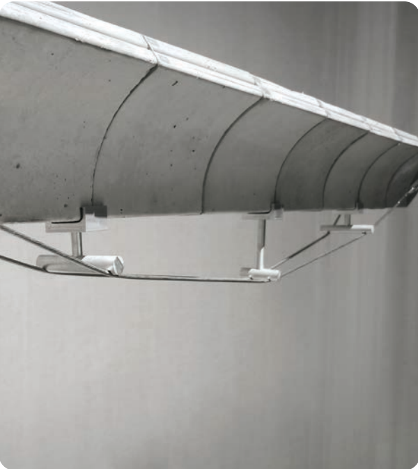
Steel tie rods on concrete bridge
